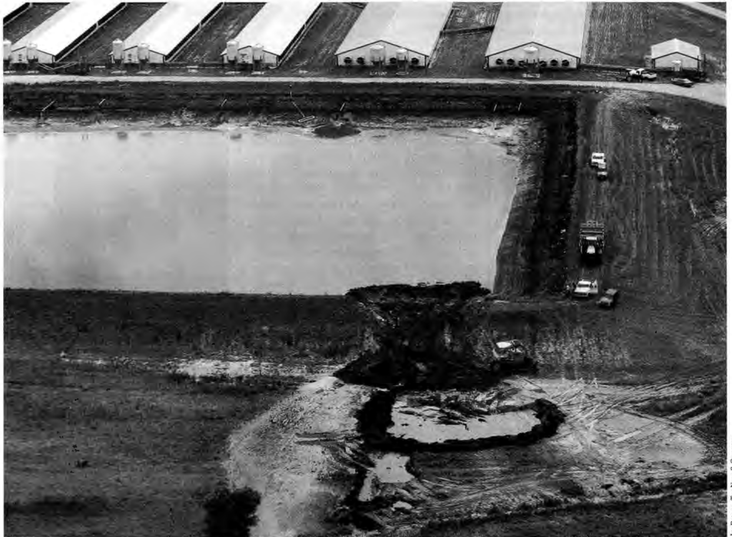
June 22, 1995: The collapse of an earthen wall sent 25 million gallons of hog feces, urine and sludge from this waste lagoon at a farm in Onslow County, N.C., into the nearby New River, causing a massive fish kill and closing down marinas and commercial fishing operations downstream.
