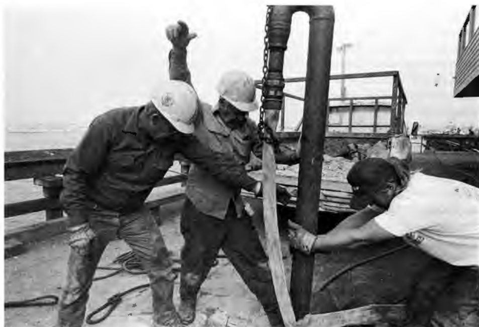
Piledrivers working at pier in Newport Beach, Calif.
