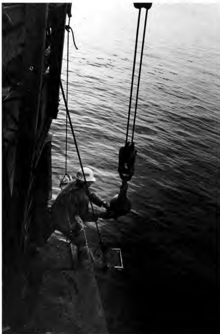
Piledrivers clearing debris at pier in Newport Beach, Calif.
