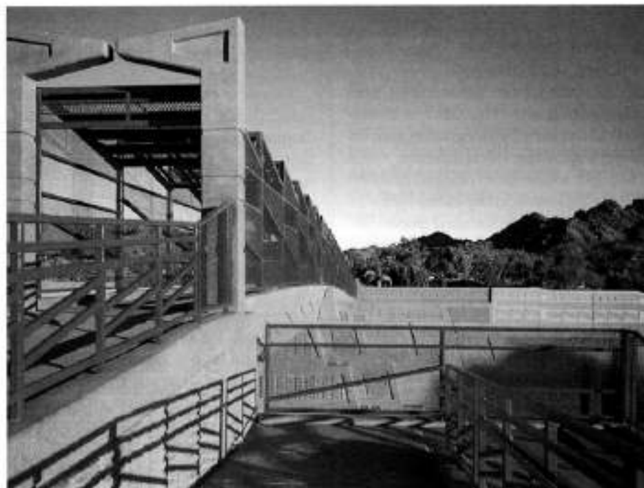
"Dreamy Draw Pedestrian Bridge," on the Squaw Peak Parkway at 29th Street, designed by Vicki Scuri.
