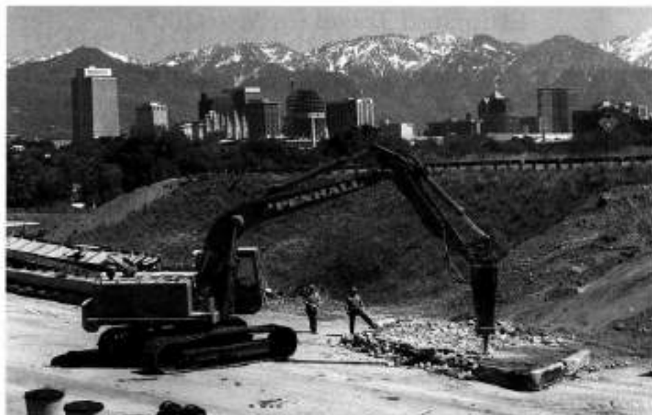
I-15 construction, Salt Lake City.
