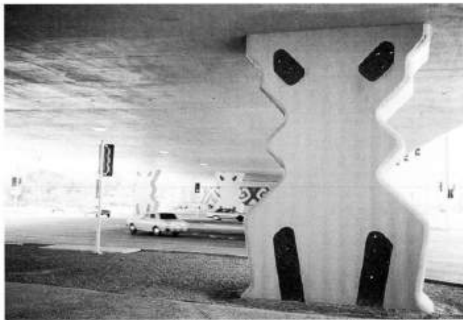
"Our Shared Environment," on the Thomas Road Overpass. For the columns holding up the bridge design team artist Marilyn Zwak made a composite of Hohokam Indian zoological forms, which typically have a triangular, diamond-shaped belly. "We would call it a frog, I suppose."
