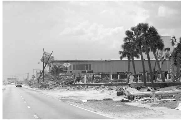
AFTER: The same stretch of U.S. Highway 90 in Biloxi taken four days after Hurricane Katrina.
