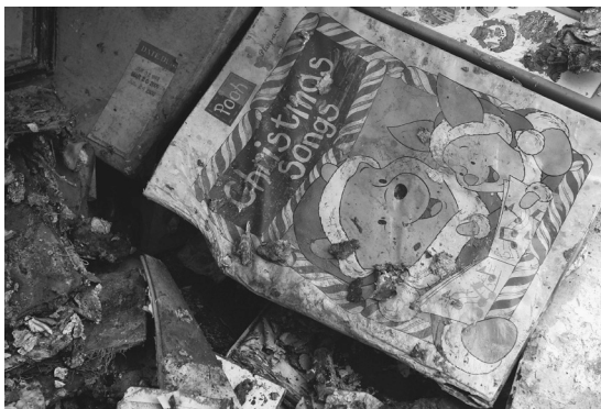
A child's book sits in the debris of a school in New Orleans damaged by Katrina. August 2006. Photo by Alex Brandon/The Associated Press.
