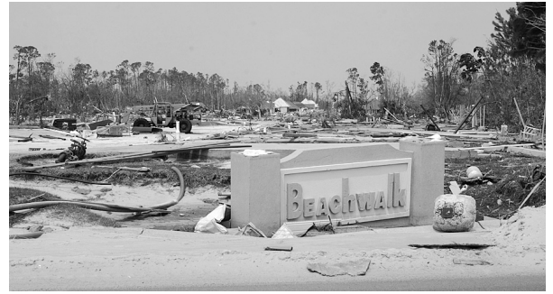
AFTER: None of the structures at Beachwalk survived the force of Katrina.
