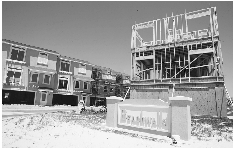
NOW: Nine months later, condominiums are being rebuilt.
