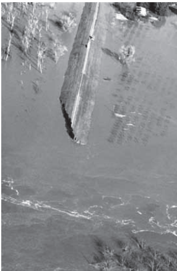
Water from the Feather River flows through a damaged levee in Arboga, California in January 1997. This break caused major damage in the region. Photo by John Trotter/©The Sacramento Bee.
