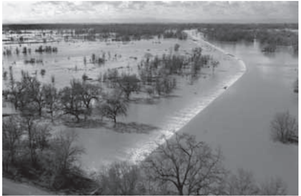
Water from the Sacramento River and Sutter Bypass flow over the Fremont Weir (distinguished by the churning white water) as it heads toward Sacramento, California in February 2004. The Fremont Weir was built in 1924 and was designed to relieve pressure from the Sacramento River when water reaches a predetermined height. Photo by Randy Pench/The Sacramento Bee.
