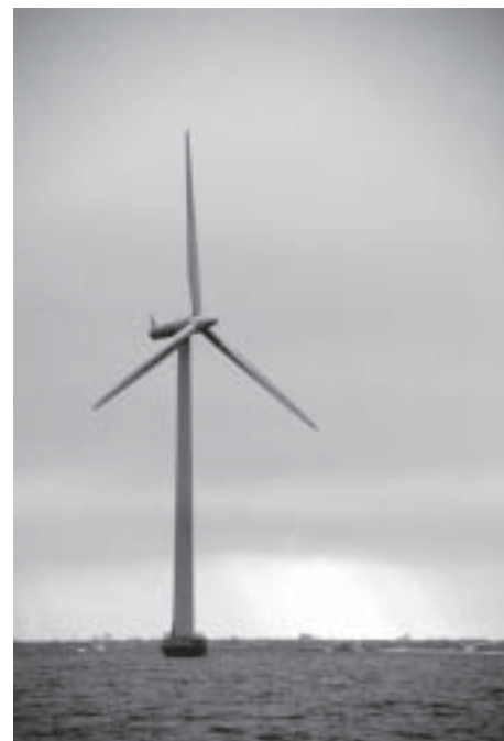
One of the 20 turbines included in the Middelgrunden Offshore Wind Farm located just outside the Copenhagen Harbor. Photo by Mads Eskesen/Courtesy of the Cape Codder Newspaper.
